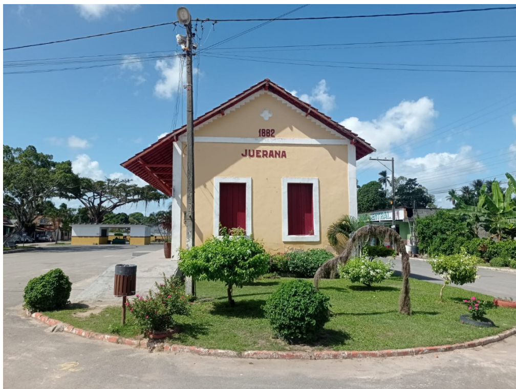
Figure 3 - Bahia and Minas Railway Station in Juerana
